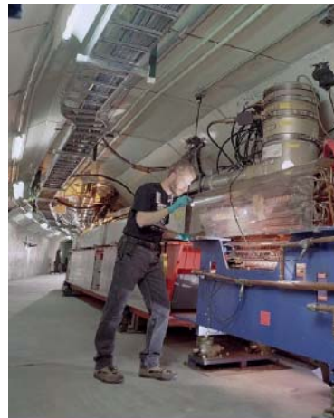
The Booster synchrotron strips electrons off H - and accelerates remaining protons up to 8 GeV
