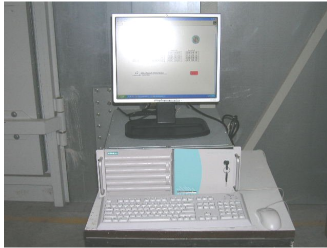
Fig. 4: Remote Control Station.
