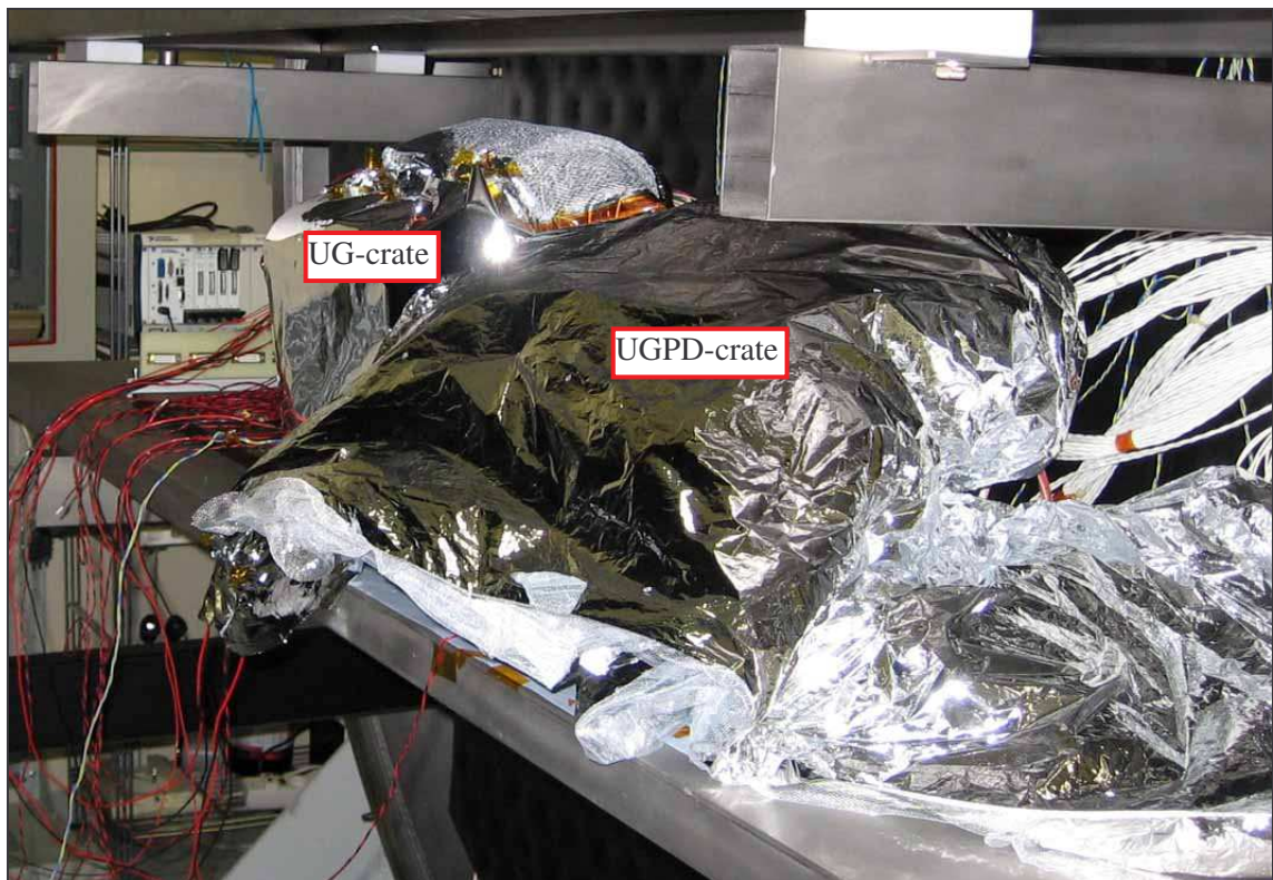
FIGURE 5 – UG AND UGPD CRATES INSIDE THE TVC COVERED WITH MLI BLANKET.
