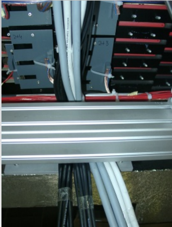
Cables to UG-crate under left Rosengitter bar
