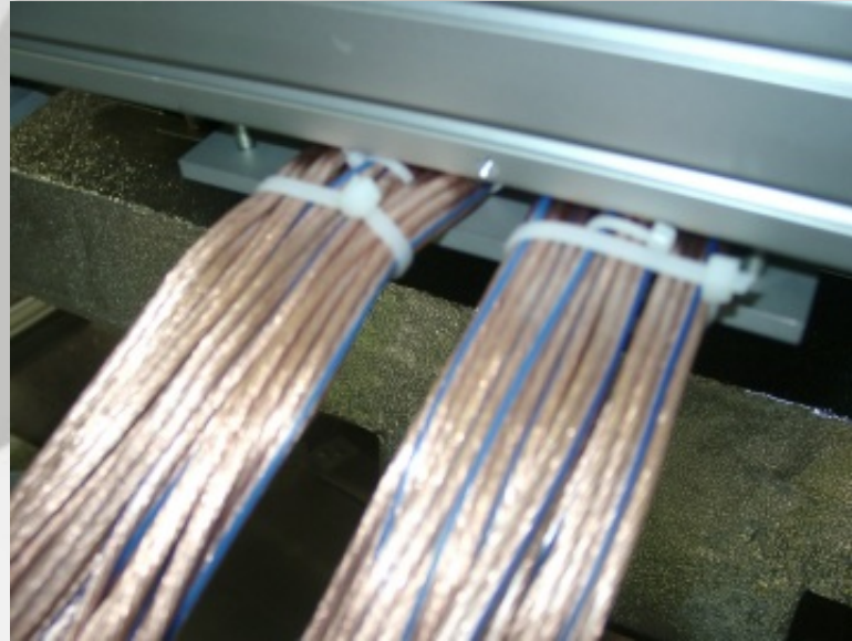
TRD-Signal cables to U-crate under middle Rosengitter bar
