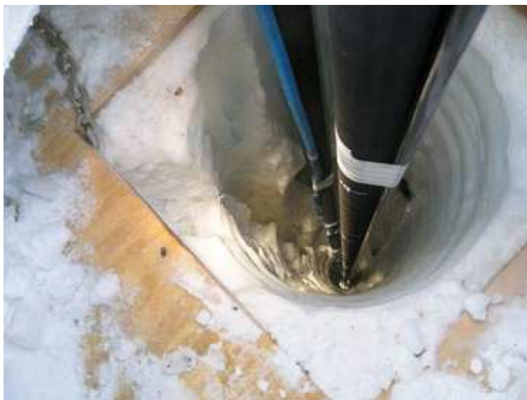
Figure 29: The hot water hose and support cables disappear down one of one of boreholes drilled into the Antarctic ice to construct the IceCube Neutrino Observatory. Photo: Jim Haugen [157]
