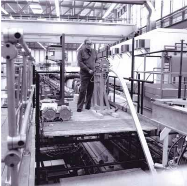
Figure 2: The pipe bringing the emulsion from the “Revolver” to the Omega target area (Courtesy of CERN Audiovisual Media Services).
