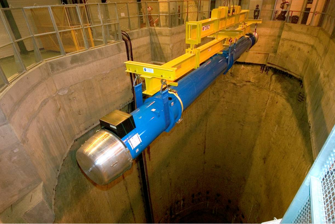
Lowering of the first dipole into the tunnel (March 2005)
