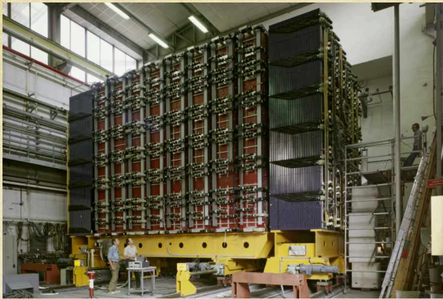
Preassembling of the UA1 magnet in the Hall 155 in August 1980. At the bottom, Peter Kalmus and Hans Hoffmann.
