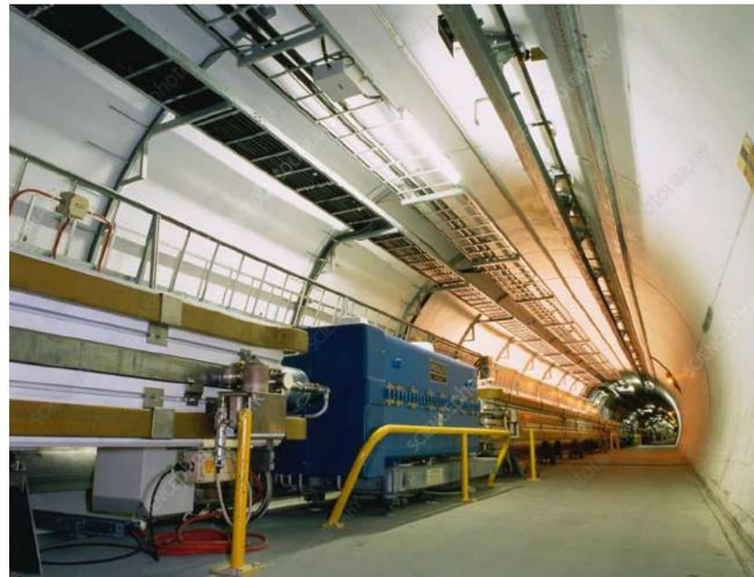
The alignment of the components of the collider was realised with a relative precision of better than 0.1 mm. The first precise measurement made with beam showed that the circumference of LEP was in fact twice as good as predicted: **better than 1 cm in 26.67 km.**
