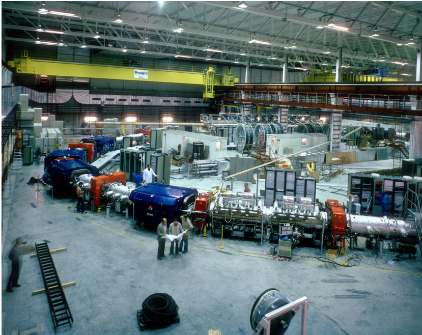
Fig. 2. View of the Antiproton Accumulator during construction.
