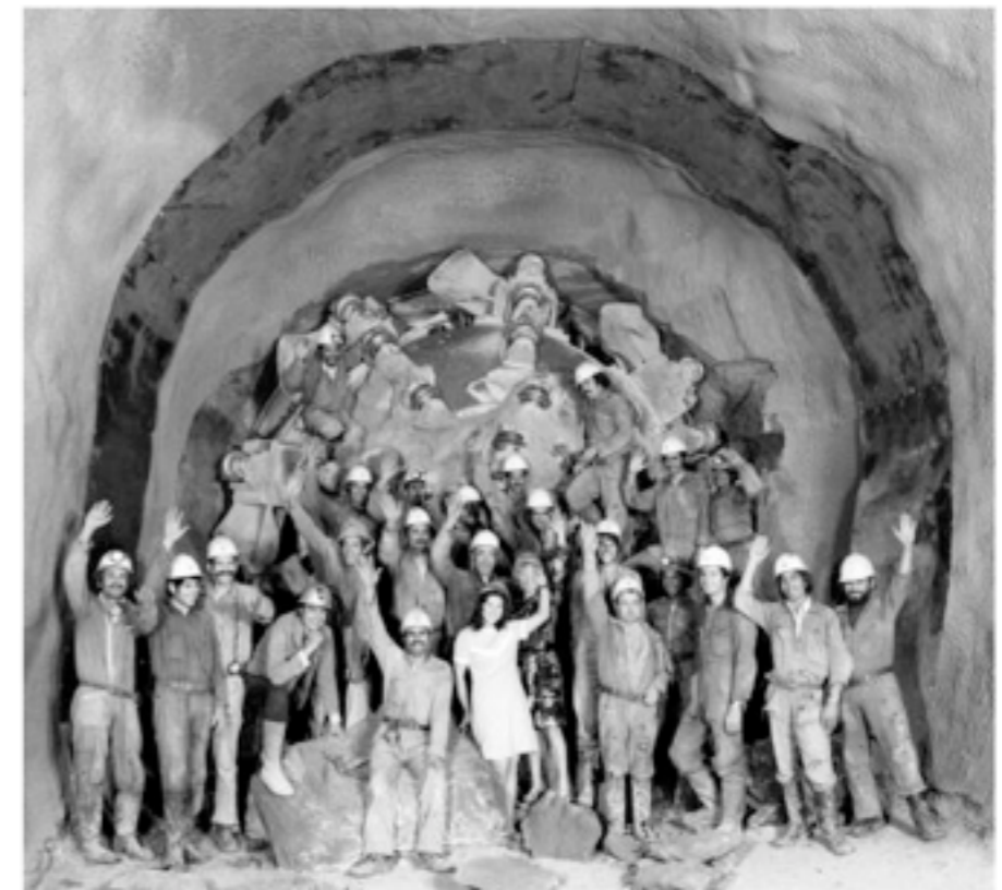
Super Proton Synchrotron tunnel completed 31 July 1974
