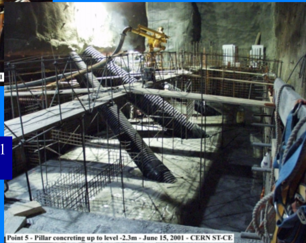
Point 5 - Installation of fibre optic ducts in the pillar (level -2.3m) - June 15, 2001
