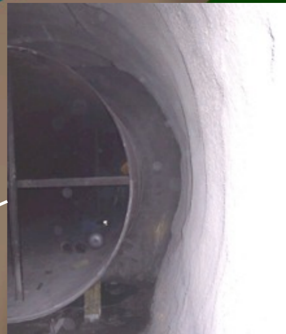
19 Nov 2003 - decay tunnel: second segment of tube installed
